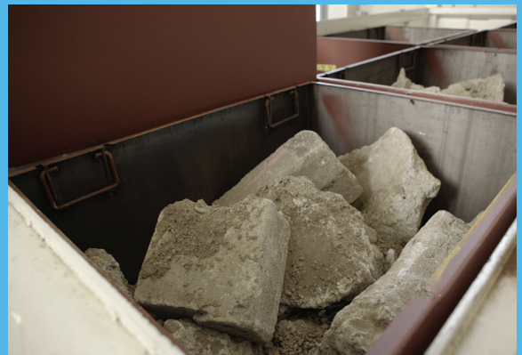
Rubble waste from dismantling
