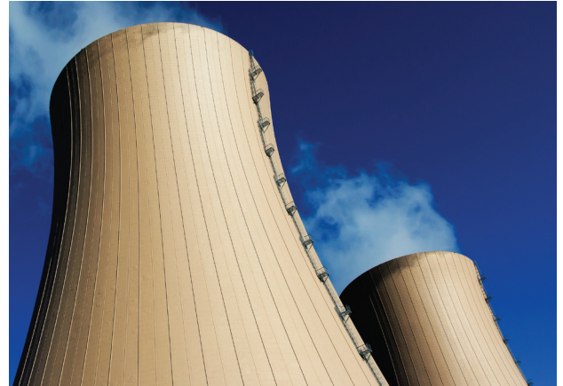
Nuclear power plant cooling towers
